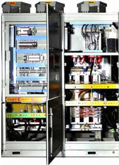
Control- and transformer cabinet
