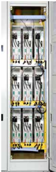
Power cells cabinet
